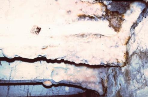
Dry Rot mycelium growing on floor joists.
